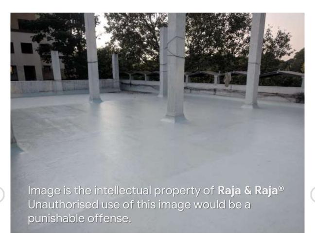
Application of the Protective top coat above the Waterproofing coating for protection from damage by traffic and UV degradation.
